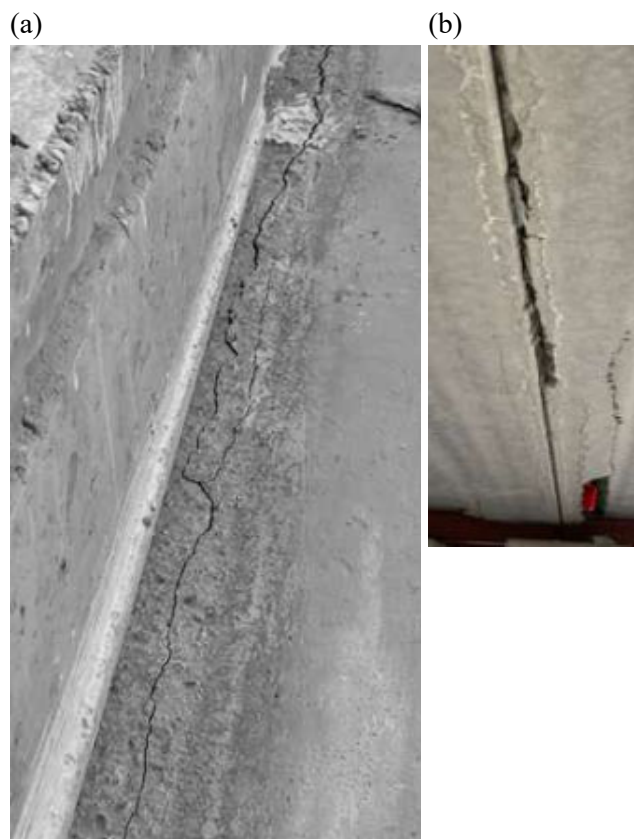
Figure 15: Longitudinal cracking (T3F2). (a) Top of floor, cracking along the grout of the joint; (b) Bottom face of floor
