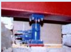
Figur 4.13 Hydraulisk demper
